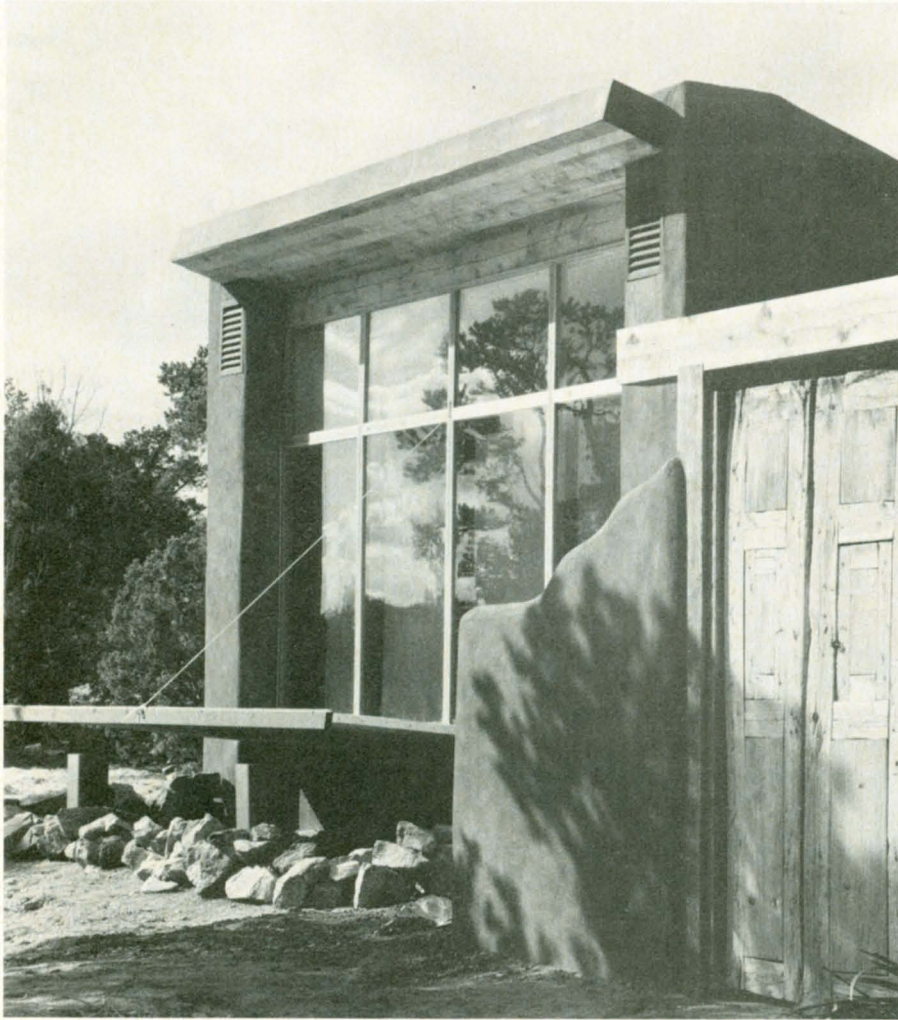
Glazed water walls store and distribute heat to the south arms of the house. Shutters, in foreground, cover the walls at night and reflect more sunlight onto them during the day.
